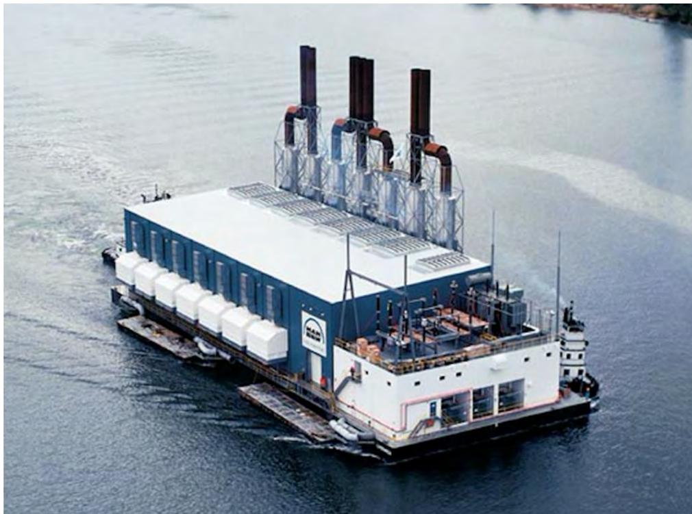
Figure 18-5: Conceptual barge mounted power plant system
